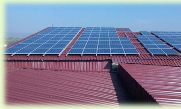
Roof Mounted Solar Panel Example (MCBÜ Köprübaşı Vocational School, Manisa)
