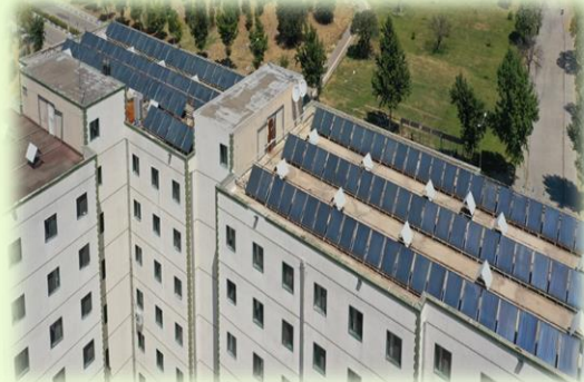
Solar Collector Example - For hot water supply (MCBU Sports Hall, MCBU Girls Dormitory Manisa)
